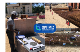
Photos : Optimiz Construction
